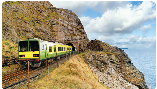
Fig. 7 Trains often use tunnels to keep the line flat.
